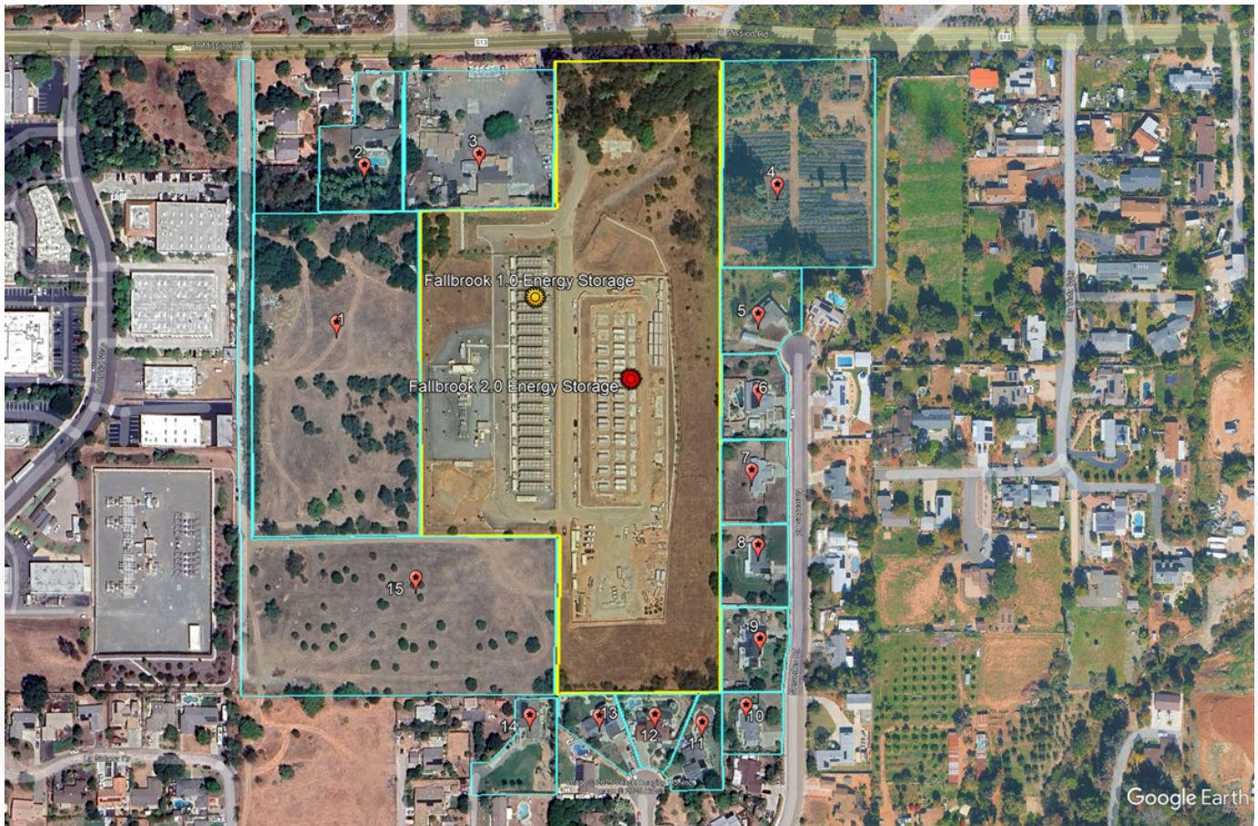
Fallbrook Battery Energy Storage System – Adjoining Properties
